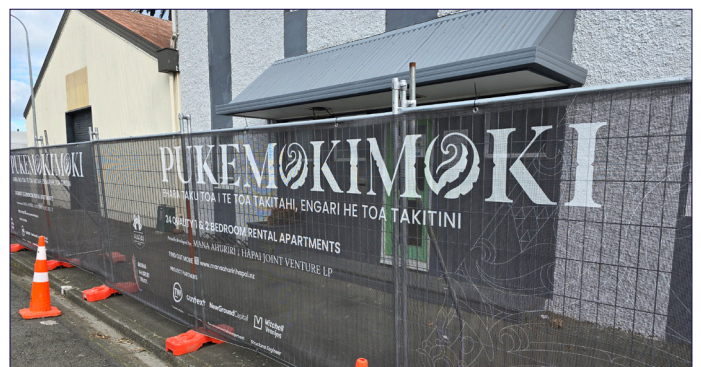
Pukemokimoki Before Demolition
