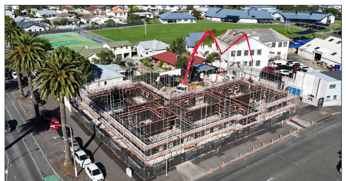
Pukemokimoki Under Construction
